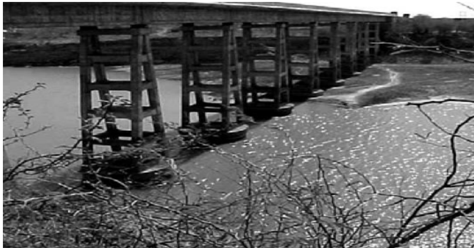
Fig 1 the Rudramata Bridge
